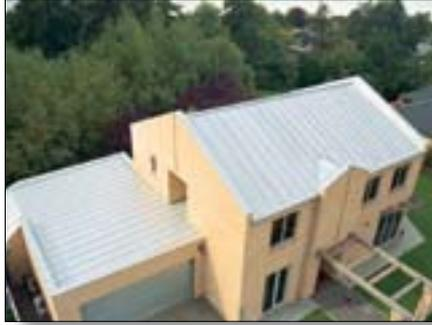
Standing-seam roofs were originally made by hand forming sheets of non-ferrous metal over long wooden boards or sarking. Crafted by skilled artisans, standing-seam roofs have stood the test of time, and to this day provide an unmistakable signature to some of the world's most beautiful architecture.
